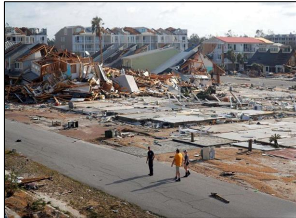
Aftermath of Hurricane Michael in Mexico Beach, FL. (AP Photo/Gerald Herbert)
