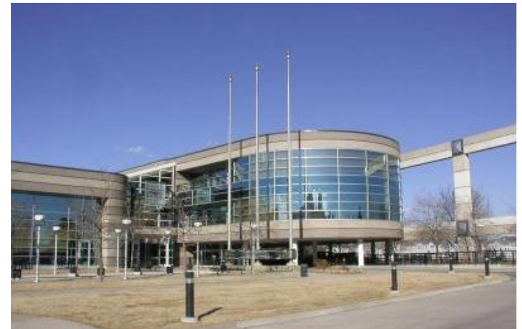
UCAR Center Green Facility
