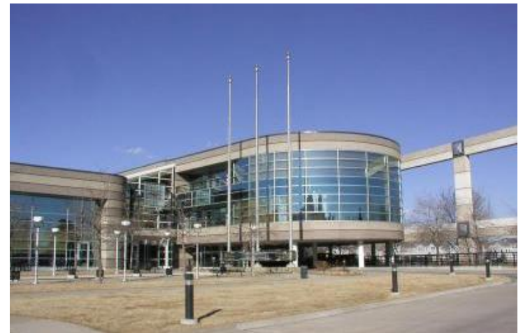
UCAR Center Green Facility
