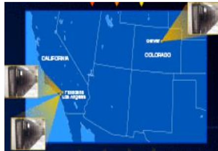
Reliable Redundant Data Centers
