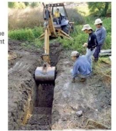
Trenching across the Hayward Fault in Fremont
