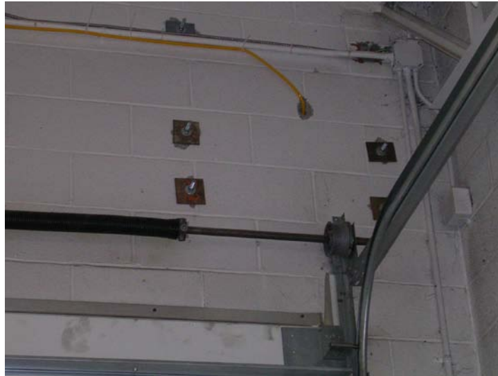
Figure 4 – Through-bolts with backing plates
