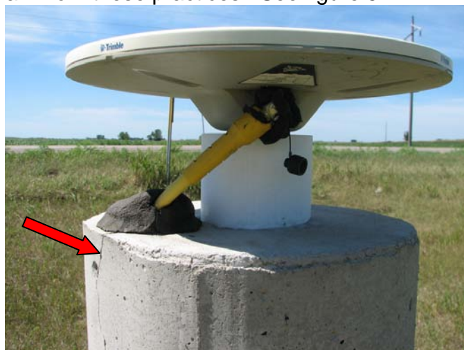
Figure 5 – view of pillar monument (note the crack that has developed near conduit location)
