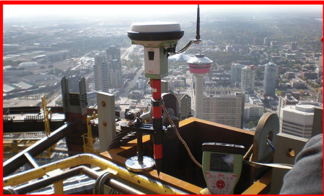
GNSS Precision Survey in construction of High-Rise Buildings
