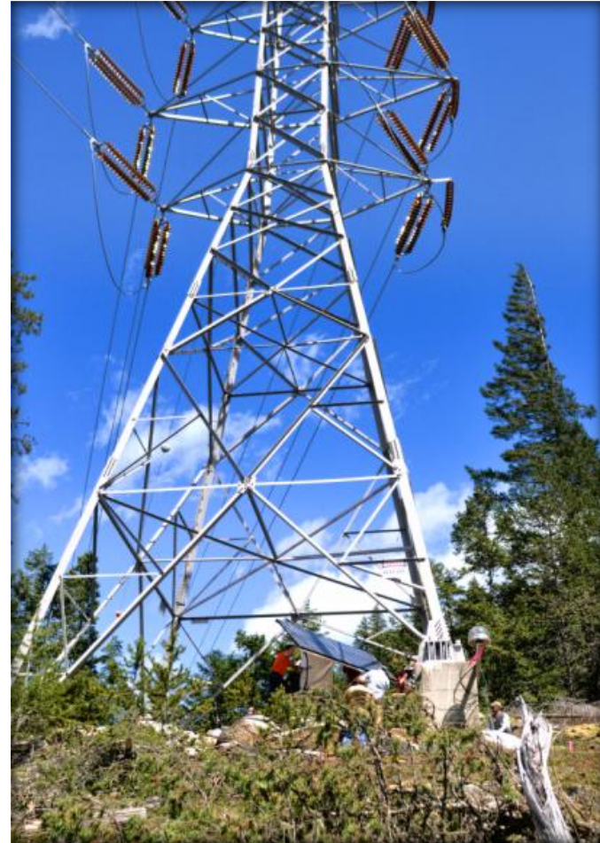
Tower Footing on Rock Promontory Monitored & Solar Array
