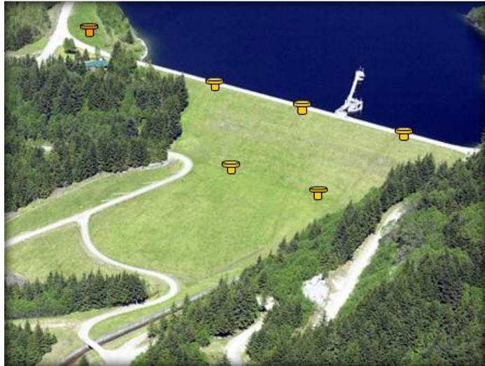
Dam Monitoring - Tolt
