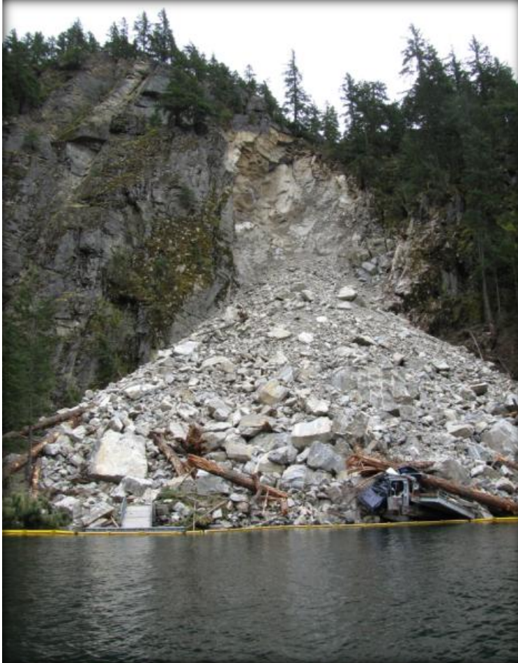
Slide – Spring 2010 Stabilization will require blasting and scaling
