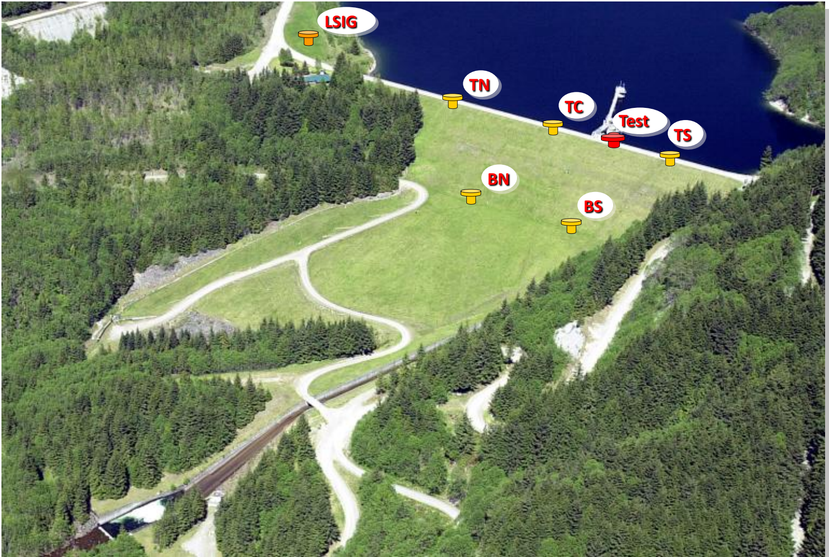
Zoned Earthfill Embankment – 61m x 300m
