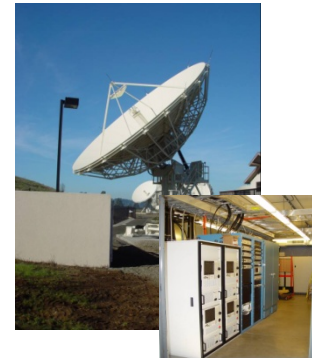
4 Ground Earth Stations
