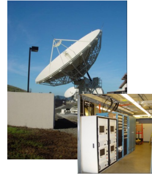
4 Ground Earth Stations
