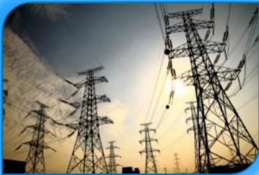
Power Grid Systems
