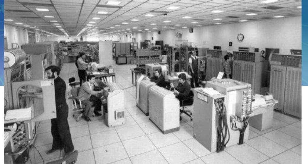
DSN Madrid wing with 642-b & 1218 computers, 1299 switches, MSFTP 2 decommutation equipment, & telemetry processors
