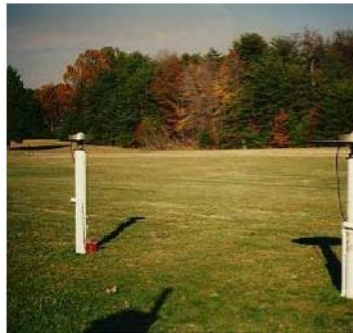
Antenna testing facility
